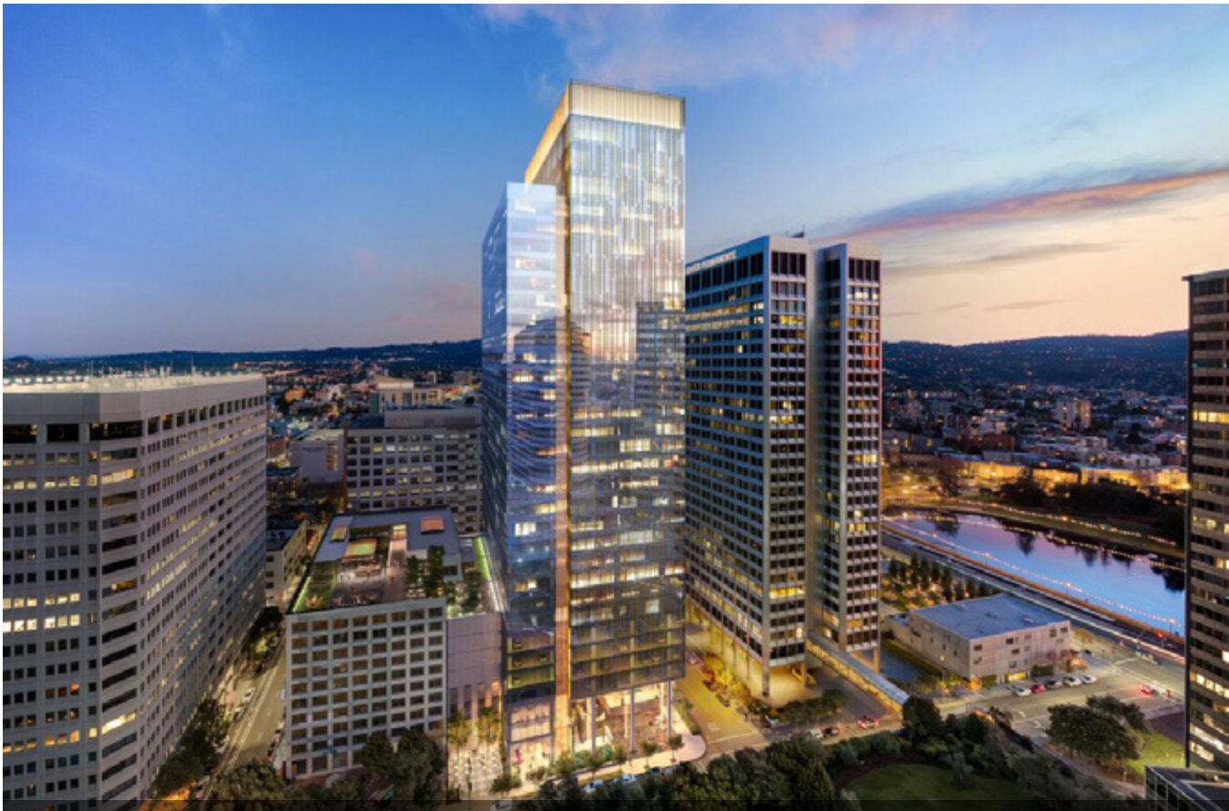
BEACON TOWER OAKLAND, CA
